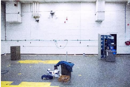
Canadian Mask Making (CMM) room preparation at the Oshawa plant to produce face masks based on the GM production model already working in Michigan.
